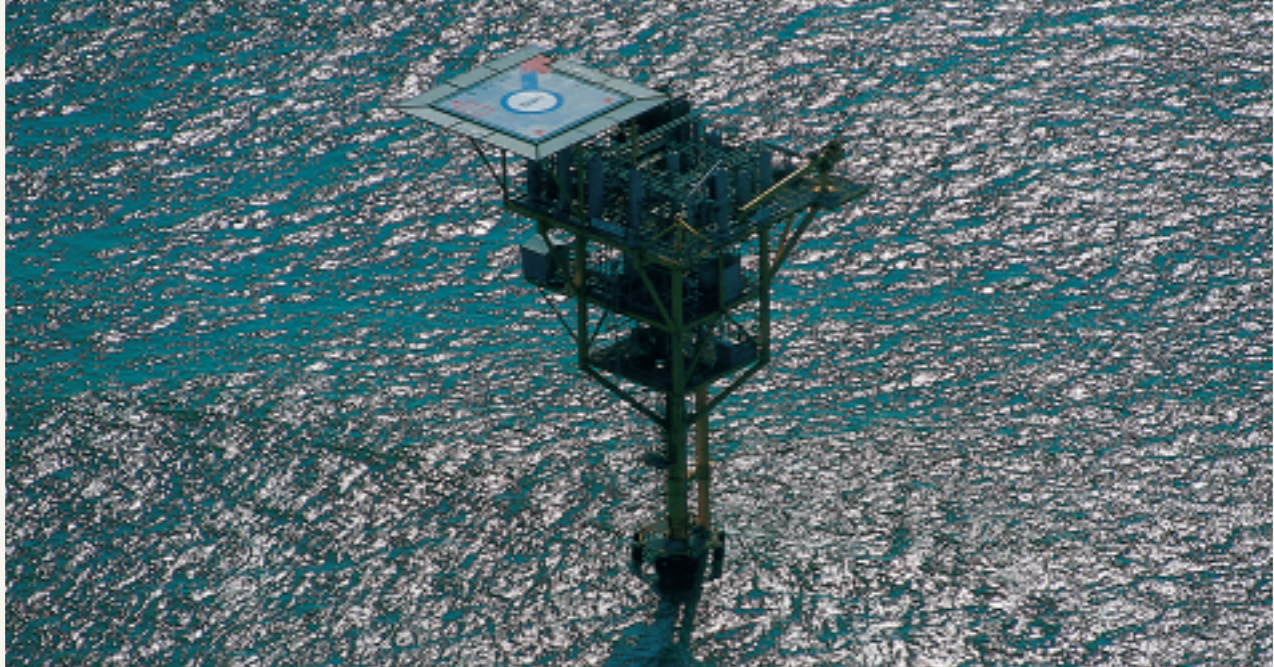
Production platform at Ship Shoal 66 B
