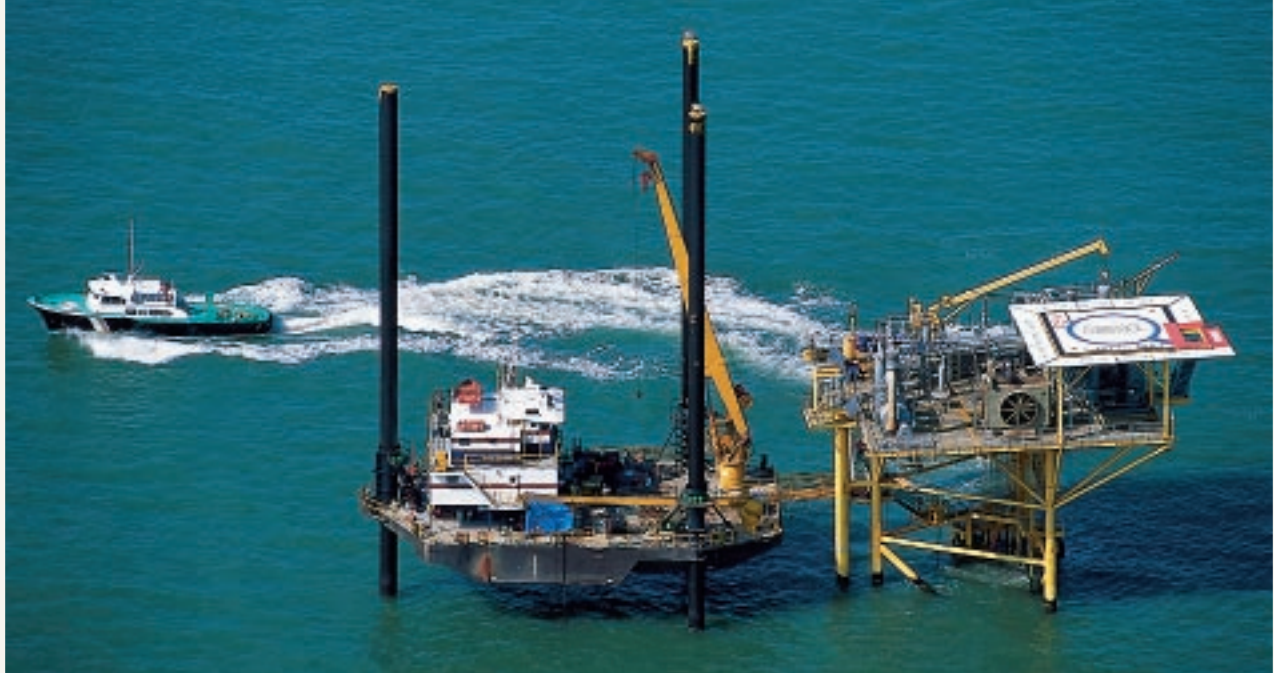
Liftboat modifying South Pelto 1 facilities for new well
